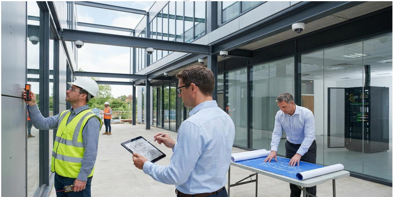
Joint site survey for camera locations, coverage and network requirements.
