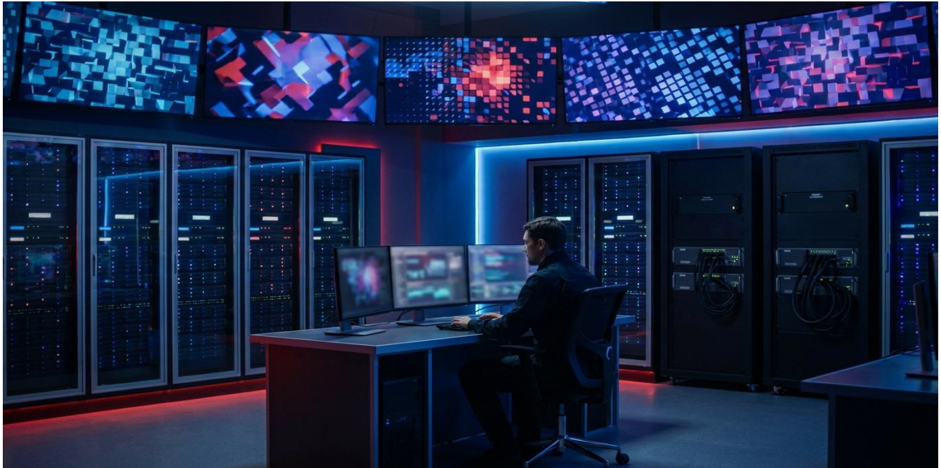
Protected VMS infrastructure with monitored, segmented network services.
