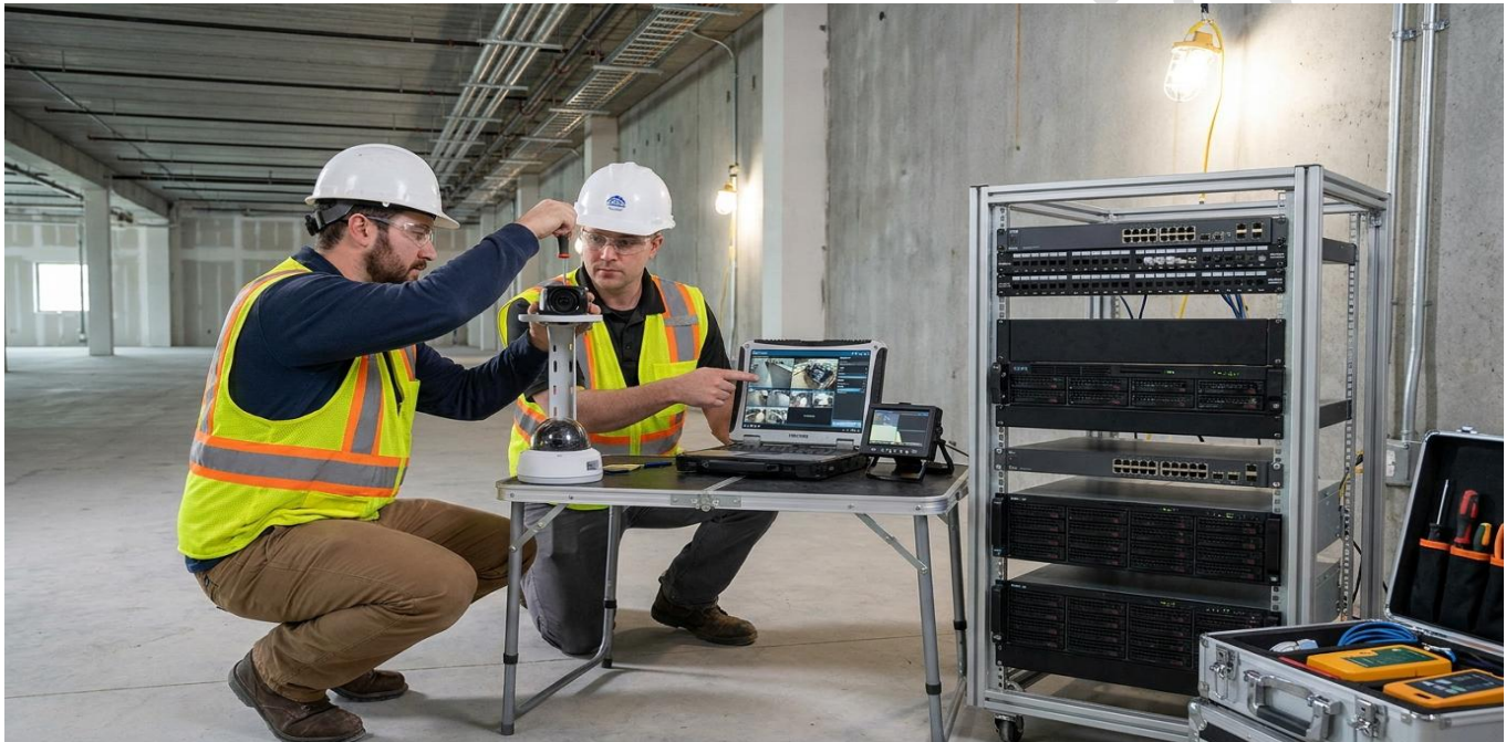
Field testing, camera adjustment and integrated VMS commissioning.
