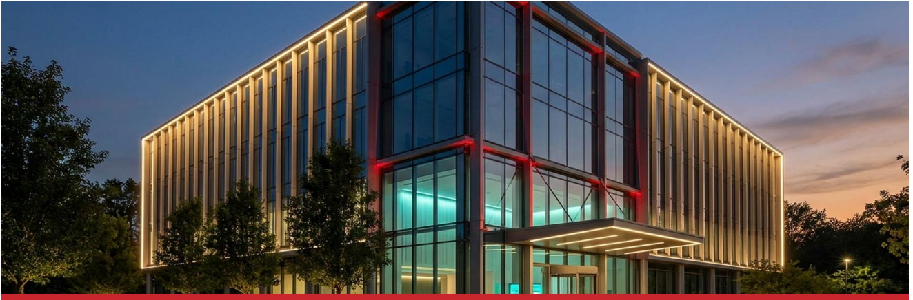
Coordinated façade, entrance, pathway, landscape and perimeter lighting
