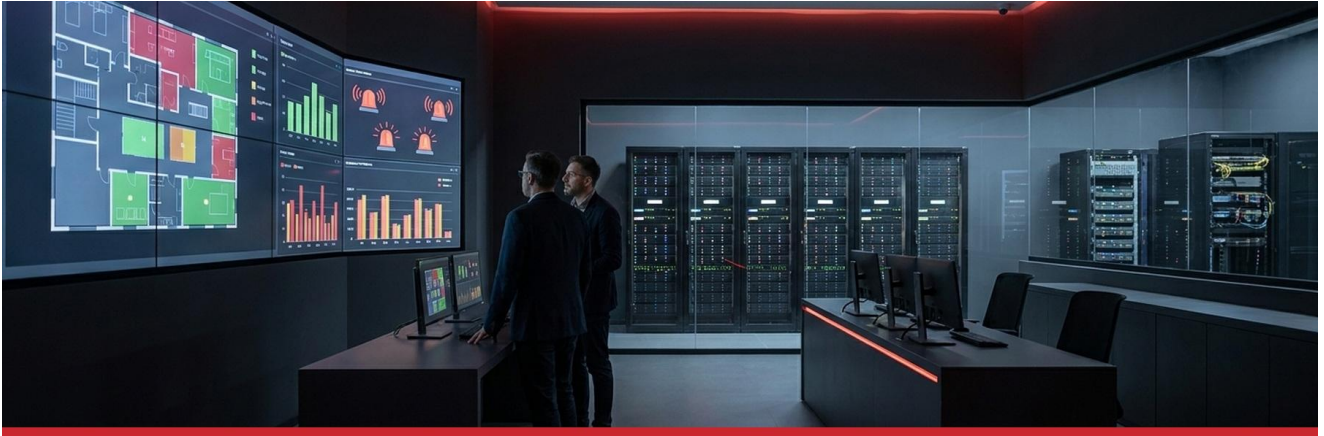
Secure head-end, server, network and third-party building-system integration
